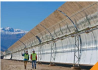
Parabolic Trough System
